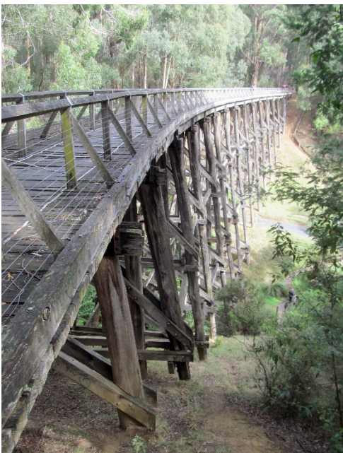
Noojee Trestle Bridge
